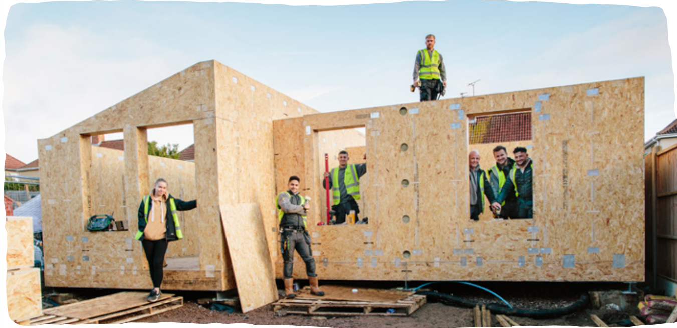
Figure: WeCanMake home build using BlokBuild system
